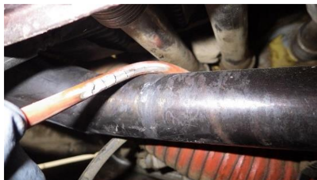
Figure 6: chafing of a high-tension ignition cable on an exhaust pipe.
