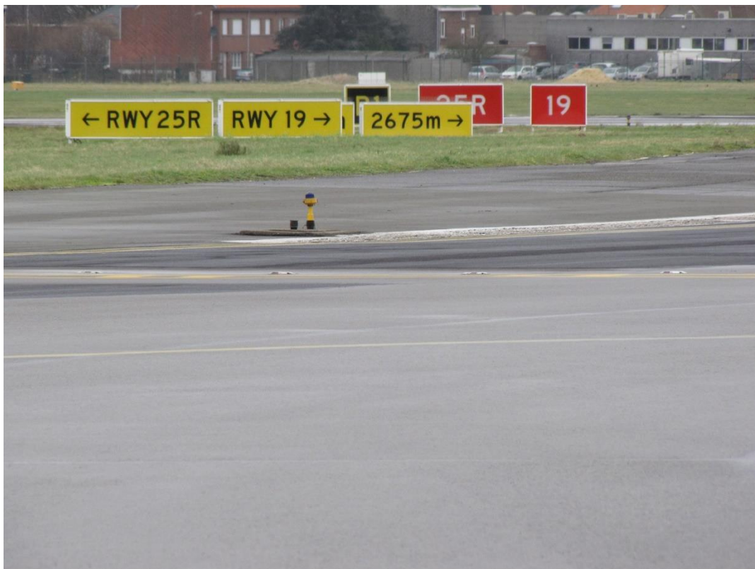
Figure 3: Holding position signs and information signs left-hand side at taxiway B1
