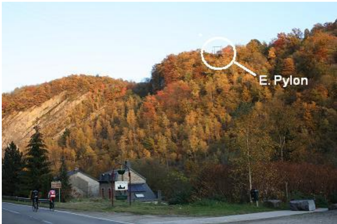
Fig. 11. HV Power line in Comblain-au-Pont.
