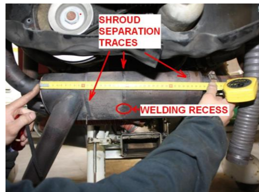
Figure 13: Traces of the shroud ribs onto the muffler + welding recess
