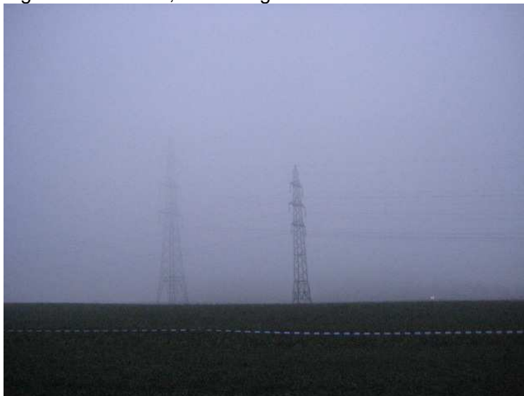
Picture taken from the crash scene (120 from the first HV line), shortly after the accident, showing the high Voltage line.
